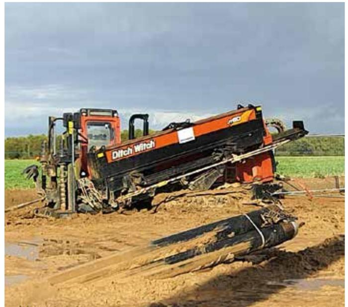
Horizontal Directional Drilling taking place on Hornsea Two
