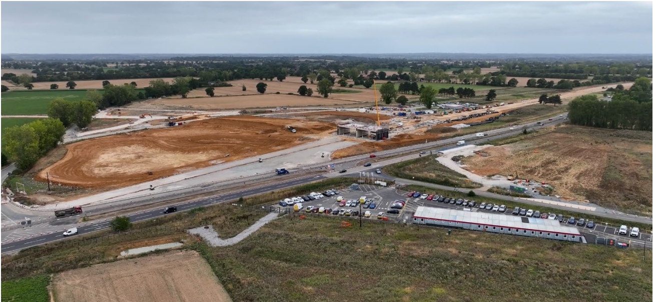
New Blofield bridge structure
