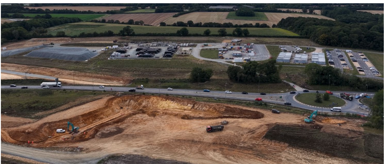
Honingham roundabout/underpass to Honingham Church
