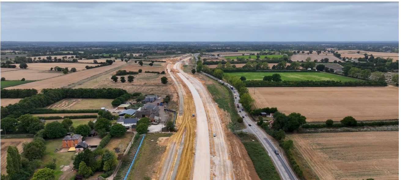
Progress of the new A47 road facing east
