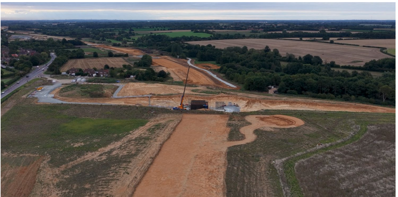
Bridge over Mattishall Lane link road
