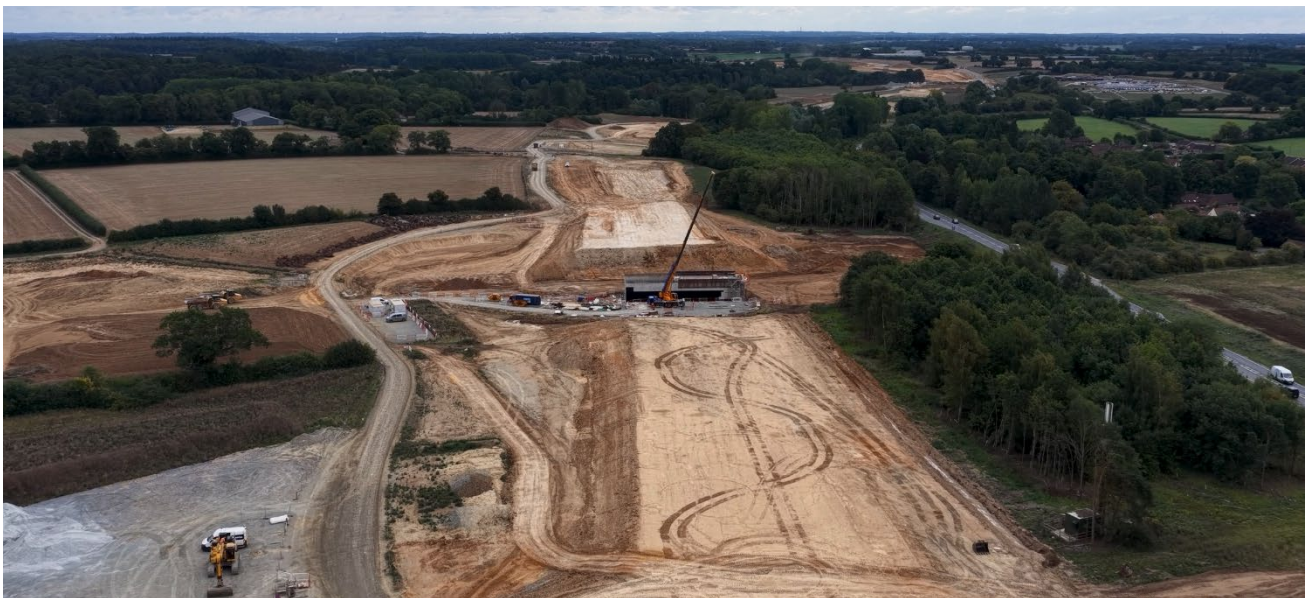
New Hall Farm underpass
