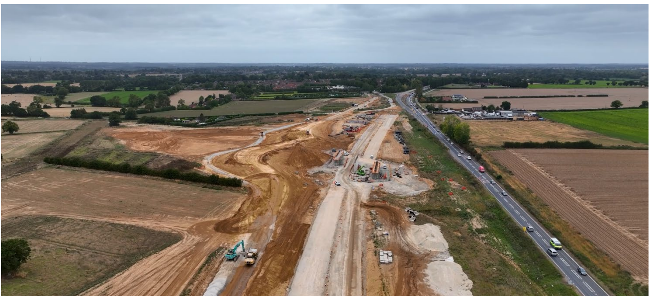
New B1140 bridge structure
